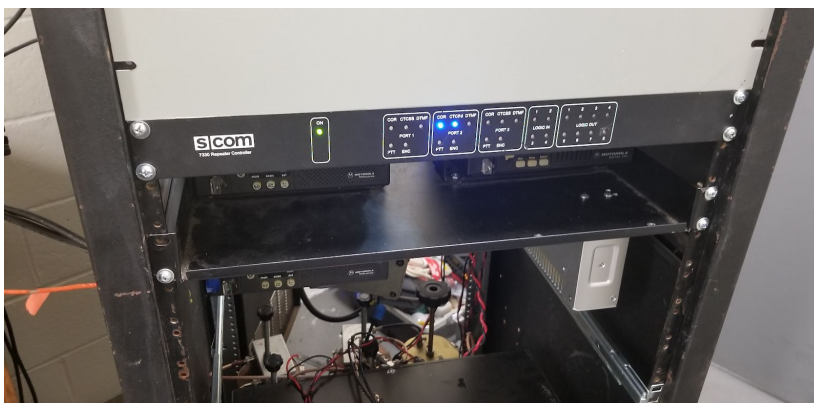
Blinky LEDs Power supply under shelf and Motorola GM300 to the left of it for 70cm control link
