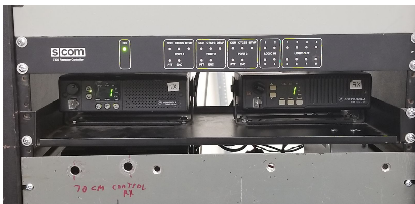
2 Motorola GM300s TX on left Receive on right
