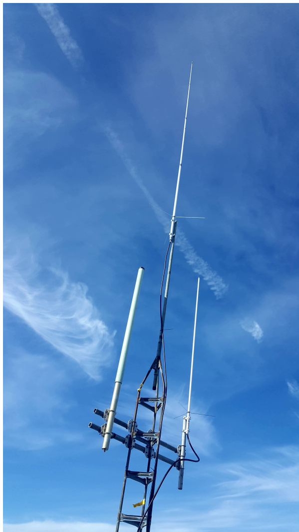
Illustration 3: The triad is complete; W1GZ's 2 meter, AB1GF's 220 MHz and W1HFN's 900 MHz antennas are now "in service." Photo KD1YH
