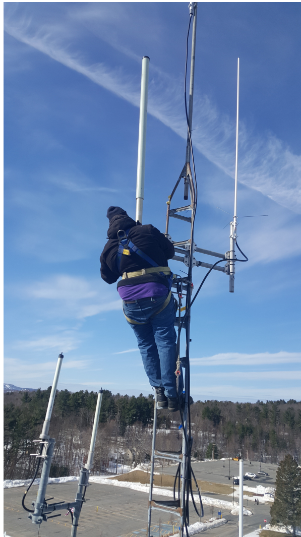
Illustration 2: MARA's resident "aerialist" AB1GF installing the 900 MHz antenna. Photo KDIYH
