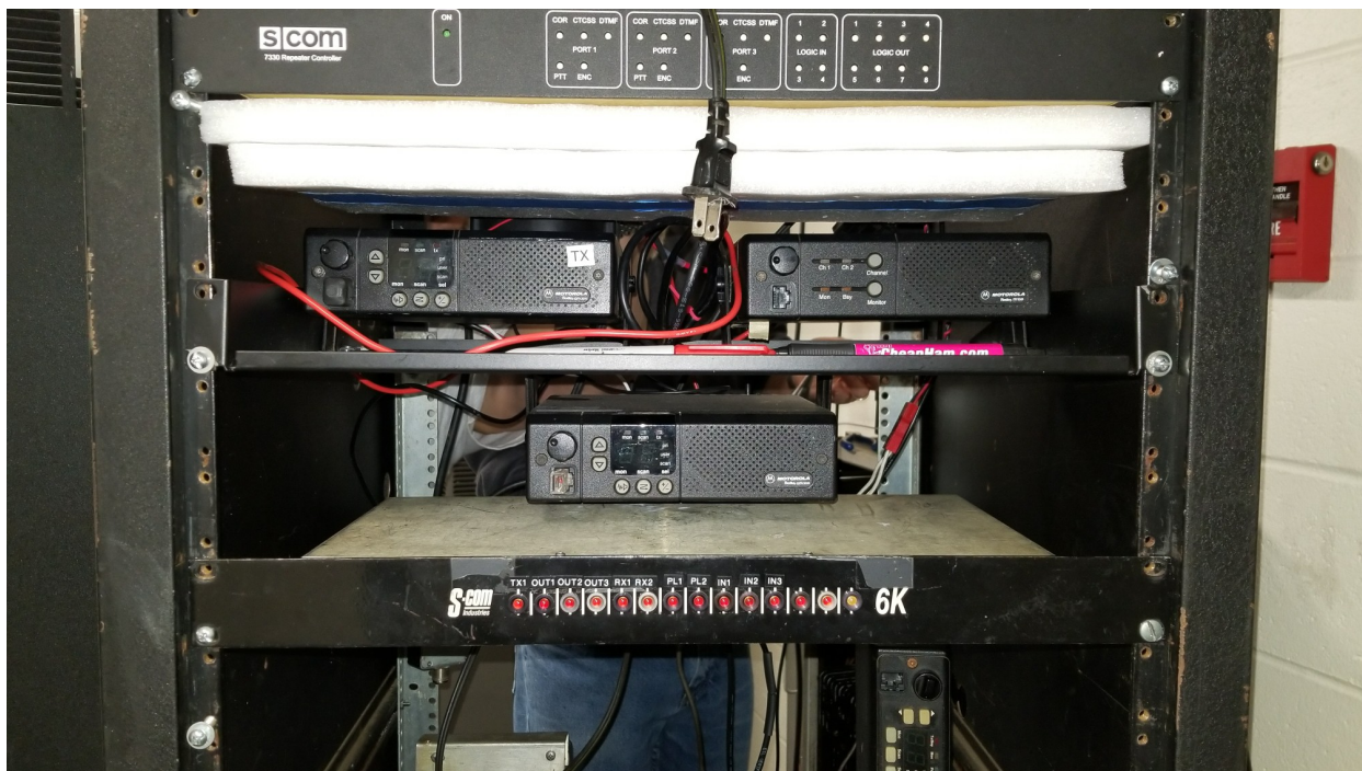
Illustration 10: Repeater equipment rack front view, Motorola transmitter, 2 Motorola receivers and SCOM controller (top)
