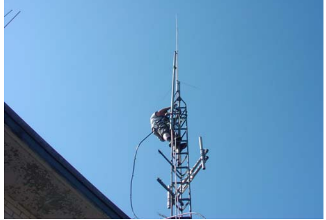
above: AB1GF strips the tower.
