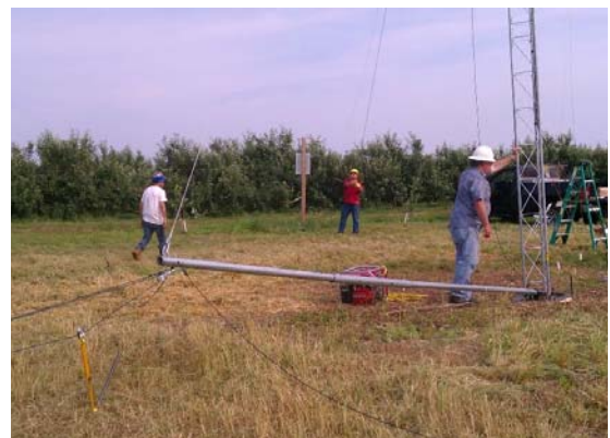
The tower is raised using a "falling derrick" method; at left the winch rope goes over the vertical pole and down to the top of the tower. At right the derrick pole is horizontal.
