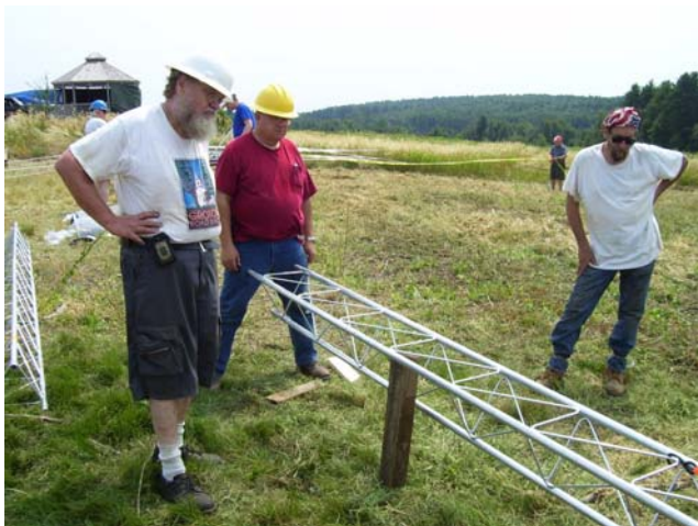
Above: Gary K1YTS, Ken KB1UVP, and Al N2KW assemble the tower.
