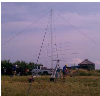
The tower is raised using a "falling derrick" method; at left the winch rope goes over the vertical pole and down to the top of the tower. At right the derrick pole is horizontal.
