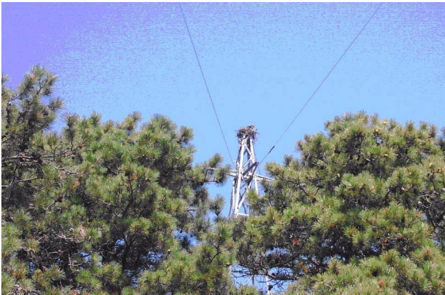
One of the still-standing 300-foot steel towers supporting one end of a rhombic. If you look carefully, you can see an osprey nesting on top.
