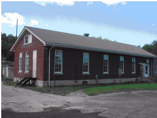
This building housed the numerous receivers and is where the ops did their thing. May be used occasionally by one of the local radio clubs for special events, although I could not get any confirmation from the ones I queried.
